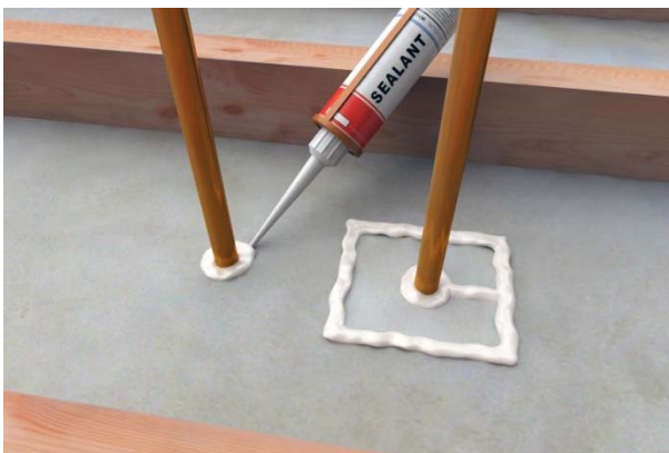
Figure 1: Sealing of Perforations Through Plasterboard Ceiling
