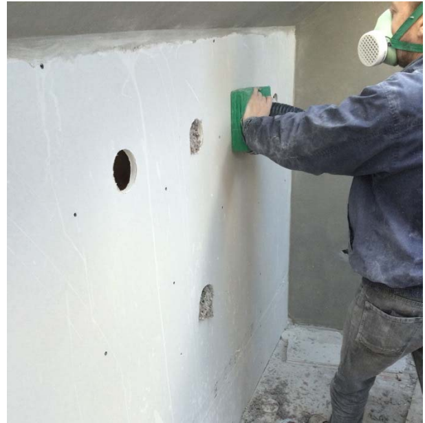
Figure 4: Operative pumping insulation into timber framed wall
